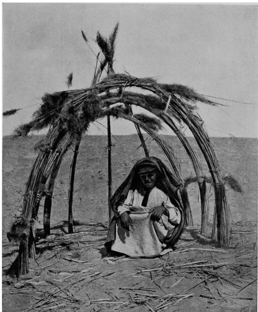
Affech Arab building a Hut of Reeds and Mats.
