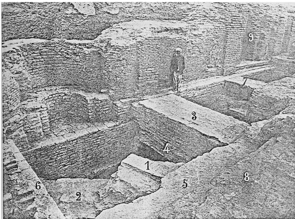
a) Sounding at Point A (seen from the North).
