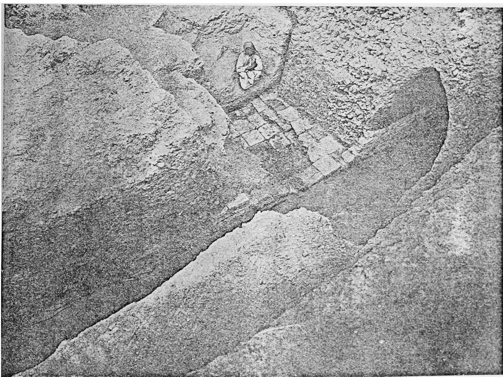
b) Shaft No. 16 (from the West).
