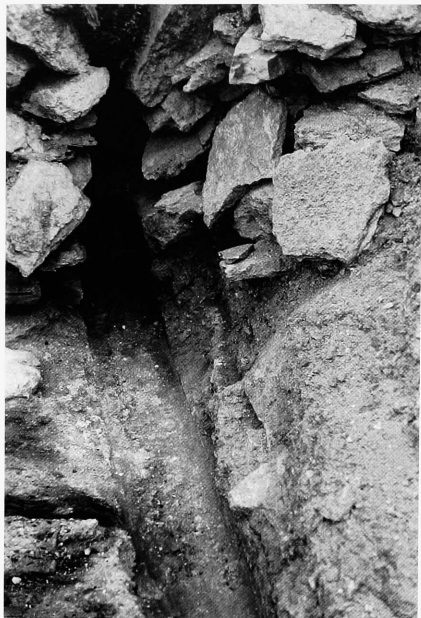
A. Tumulus S-1. Line of side wall beams extending beyond end wall in north corner. Viewed from southwest.
