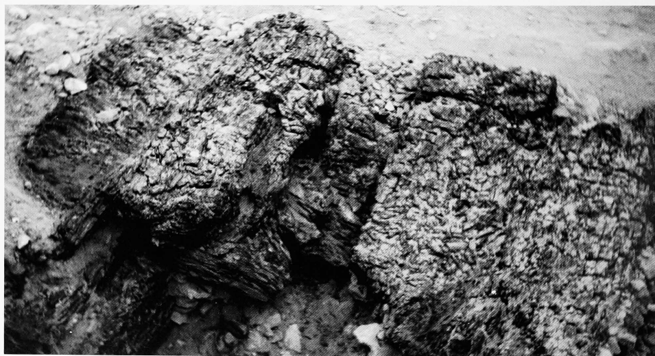
B. Tumulus G. West end showing crossing beams of double roof. Viewed from northeast.
