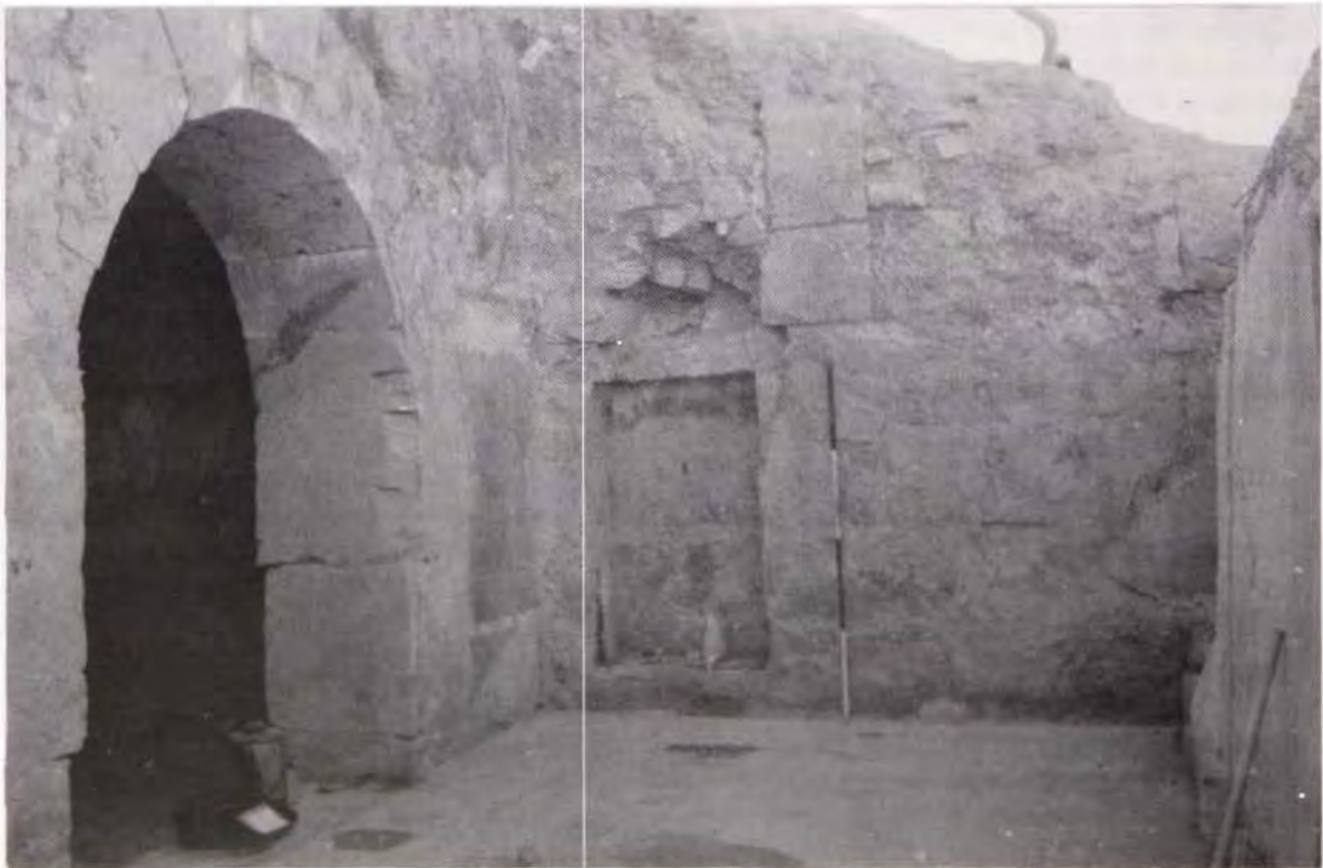
Fig. 5.5. Arched doorway into Area 3, looking NW. Note the large niche (B in fig. 5.3) in the N wall of Area 2.
