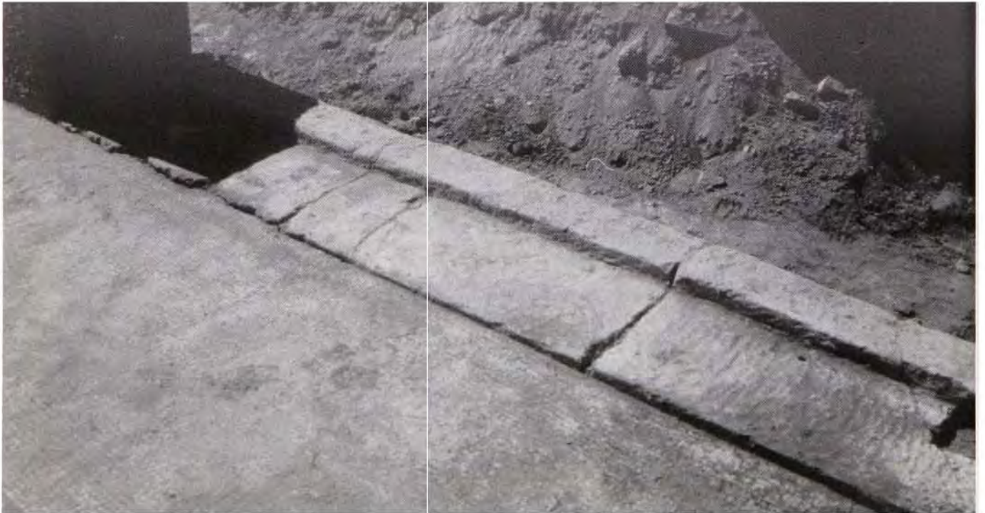
Fig. 4.6. Site D: threshold of doorway through W wall of Room 1 (mosaic room). Note rebate for the door and sockets at the right end for the door to pivot.
