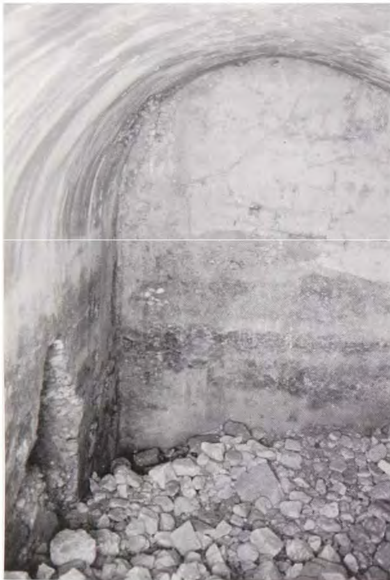
Fig. 3.11. The large cistern near the theatre
