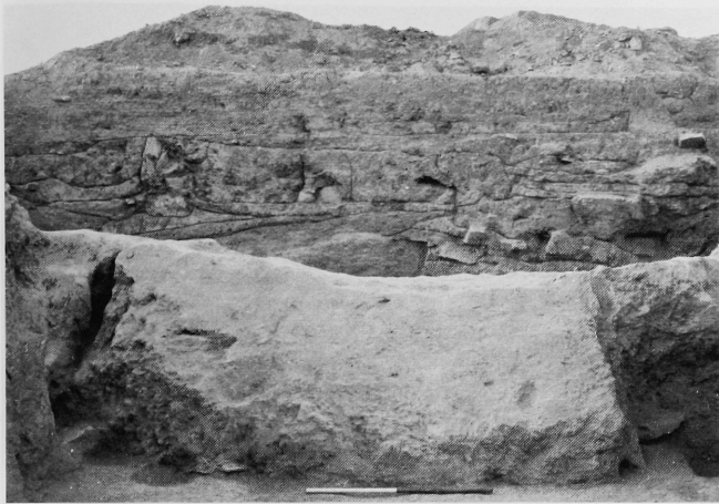
Plate IV: Evidence of the earthquake which destroyed Level III 2 : the section of wall between room 8 and area 4 which had sheered off from its foundation at floor line, split vertically at the mid point in its thickness, and slid forward from the bottom into room 8 without actually falling over (v. also wall between points A and B, Fig. 14).
