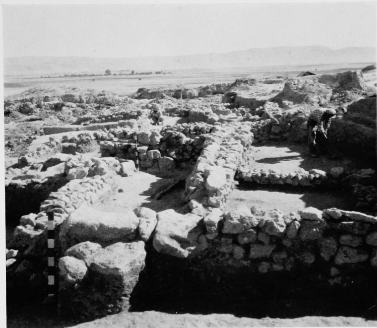
(a) Stone substructure of houses at Levels IIIa and IIIb on the eastern summit
