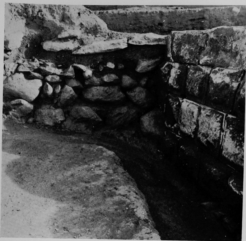
a 石壘遺構とレンガ壁接合部 Stone wall and sun-dried brick building
