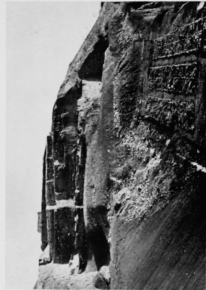
d. Foundations of Halafian fortifications at Level XVII
