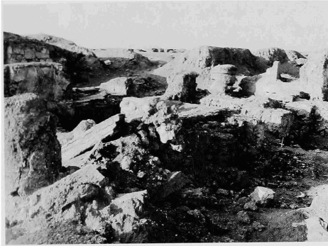
Fig. 2. View of portico in room 5 before start of work in 1992.
