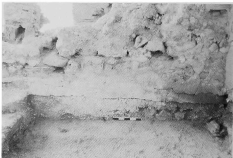
Fig. 13 - North wall of pronaos-naos 11-16 at end of excavations in 1992.
