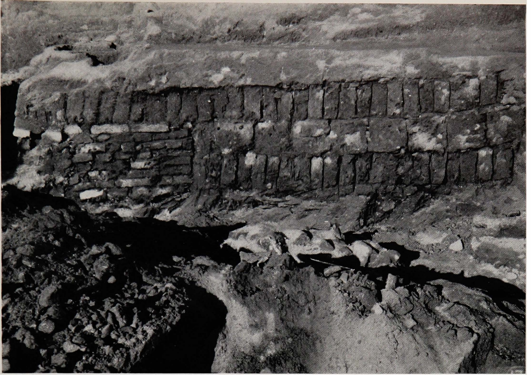
FIG. 1. Foundation structure under northern end of Court 205, Level II, looking north
