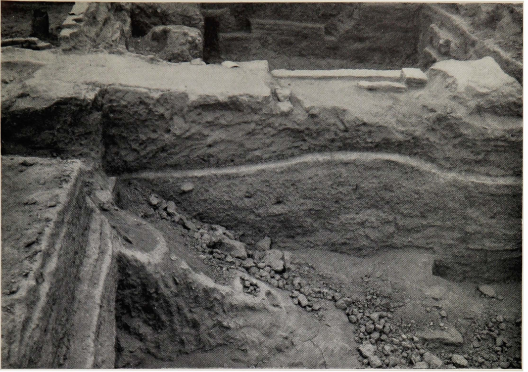
FIG. 1. East wall of Room 22, Level III, showing uneven settling of foundations under door
