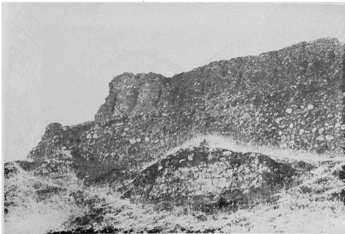
(b) Site no. 89, east section. with arrowslits.
