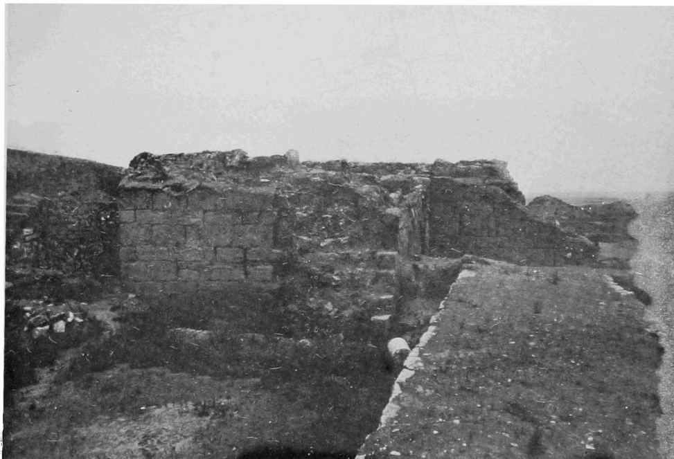
(b) Tower of the inner wall, northern gate, Hatra.
