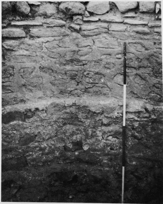
28. K21. Wall 1, inner face (CP 1 & 2). View NNE. Scale: 2 m.
