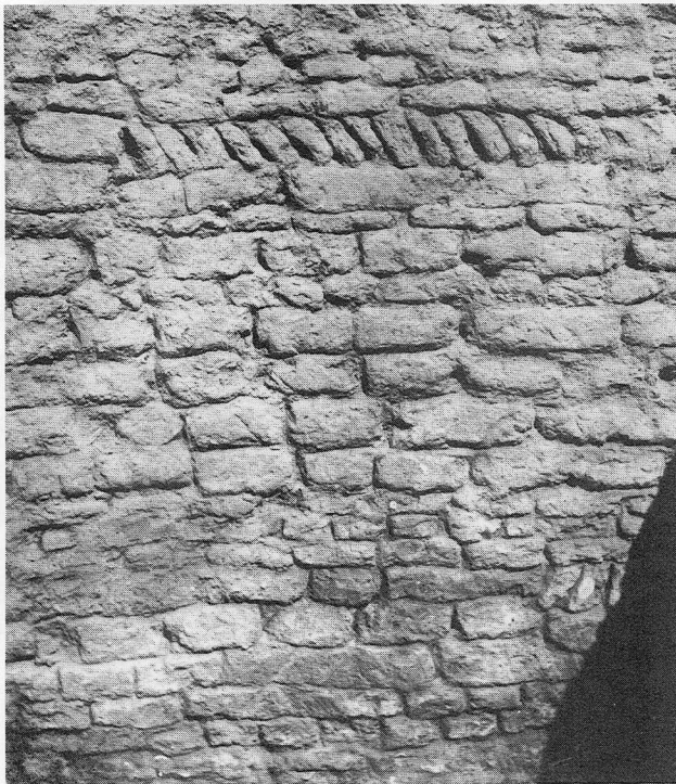
c. Ziggurat terrace. A wall of the Archaic II building built with mud bricks of different sizes and shapes, both flat and plano-convex.
