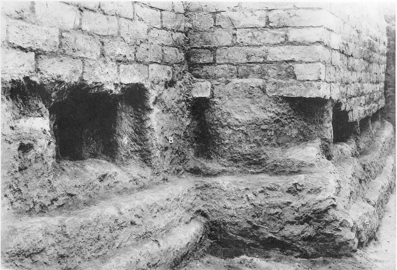
b. The E. corner of the Nannar courtyard: the outer wall-face showing: A, the burnt-brickwork of Kuri-Galzu; B, the half-column construction of Warad-Sin; and C, earlier foundations. (See p. 82)
