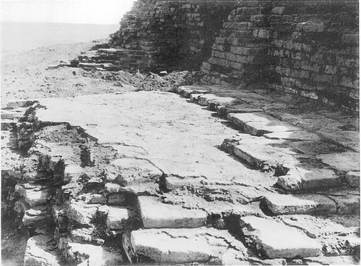
a. NW. side of Ziggurat, upper terrace: Nabonidus' pavement and retaining-wall of upper staircase, view looking NE.
