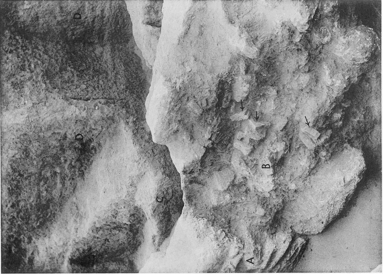
b. NW. retaining-wall: A, stone face, and B, stone core of Archaic I wall; C, mud-brick wall of Archaic I; D, mud-brick wall of Archaic II. Arrows show burnt plano-convex bricks mixed with the stonework. (See pp. 1, 8)
