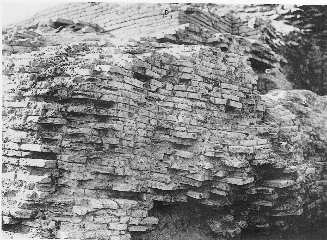
a. The SE. side of Taylor's cut, showing: A , brickwork of Ur-Nammu, the S. corner of the gate-tower; B , upper staircase wall of Ur-Nammu; C , pavement of Nabonidus; D , upper terrace front of Nabonidus
