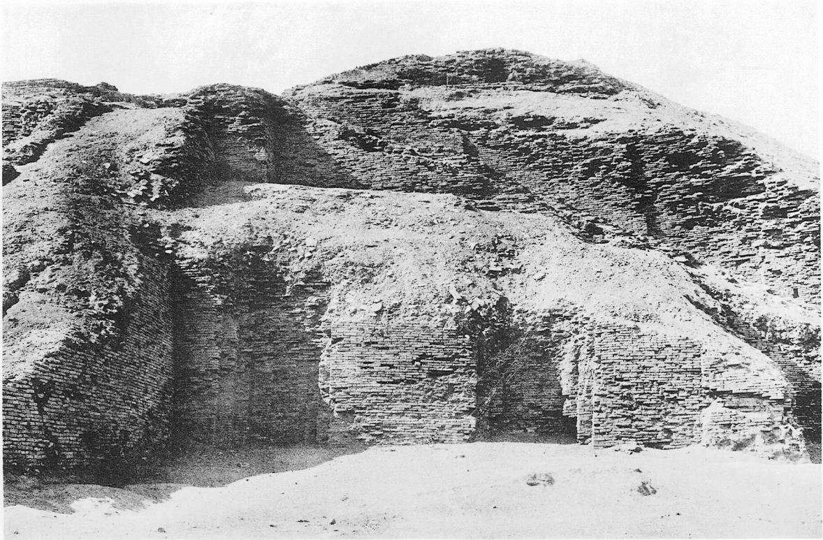
b. The NE. face: the NW. buttress in the stair-angle
