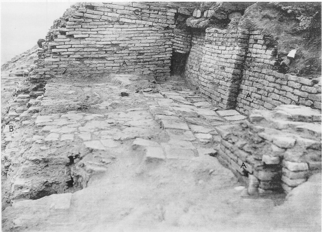
b. The terrace chamber: A, A, A, Ur-Nammu walls; B, Ur-Nammu wall-foundations; c, later brickwork. (See p. 110)
