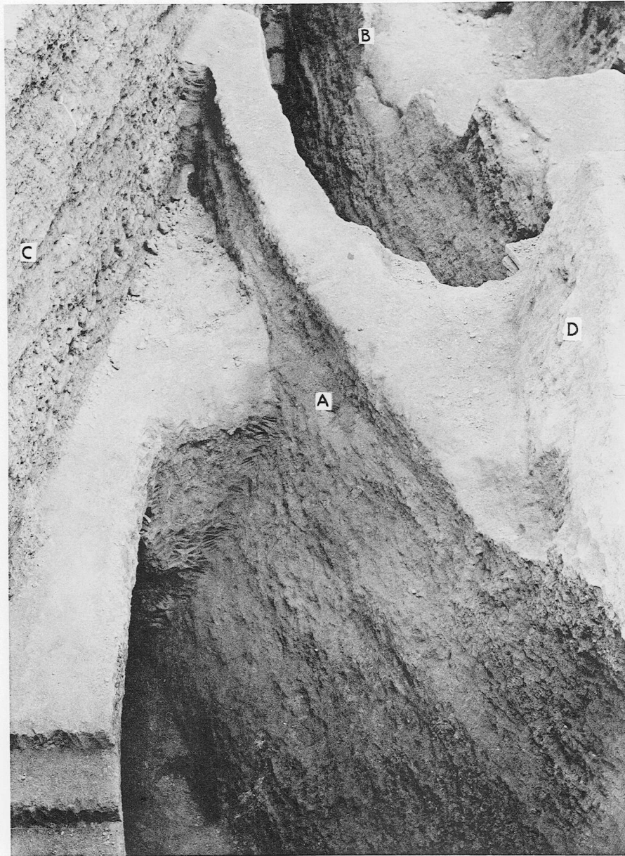
a. A, revetment-wall, Archaic IV; B, terrace wall, Archaic III; C, terrace wall, inner face, Archaic II; D, upper platform, Archaic II B. (See p. 5)
