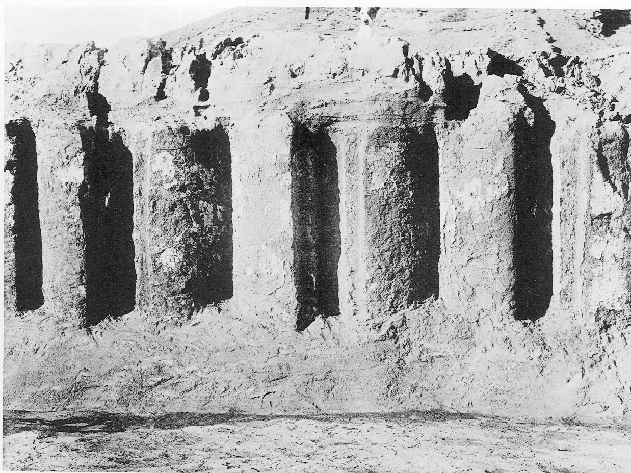
b. Detail of the SW. mud-brick wall, showing traces of whitewash. ( See p. 89 )
