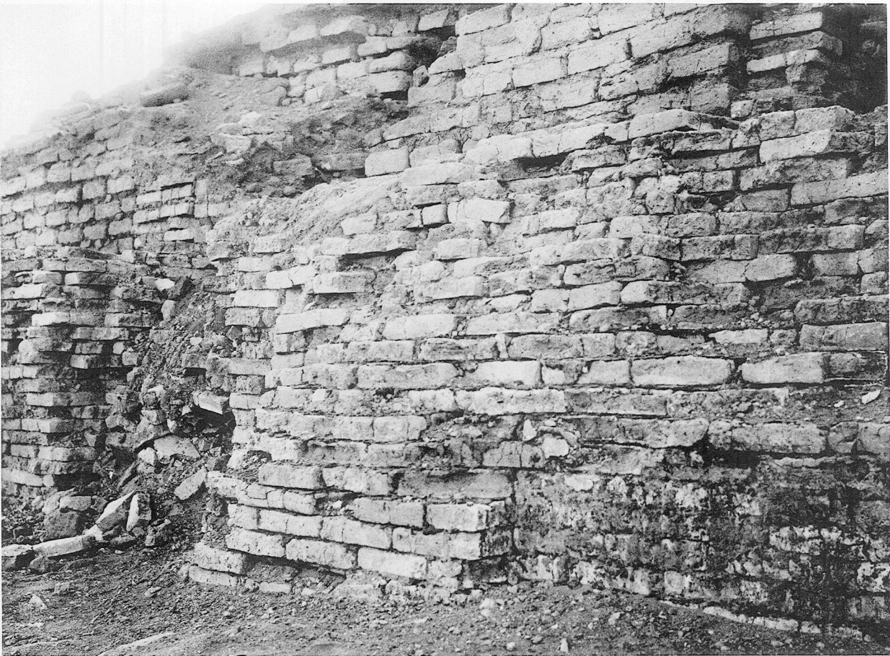
b. The same: the retaining-wall of Nabonidus, showing buttress. ( See p. 127 )
