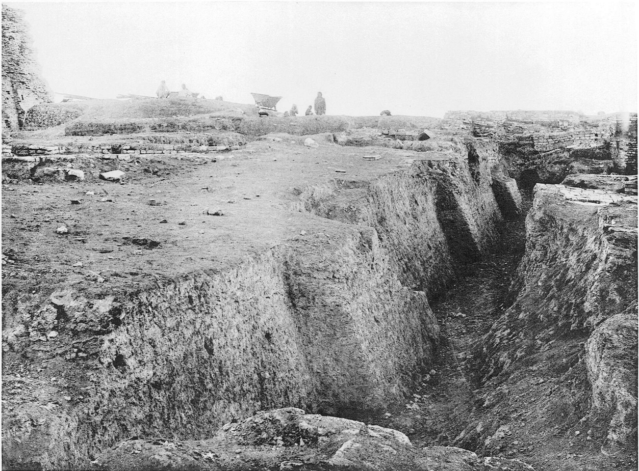
b. The terrace wall of Ur-Nammu, NW. side: general view. ( See p. 24 )
