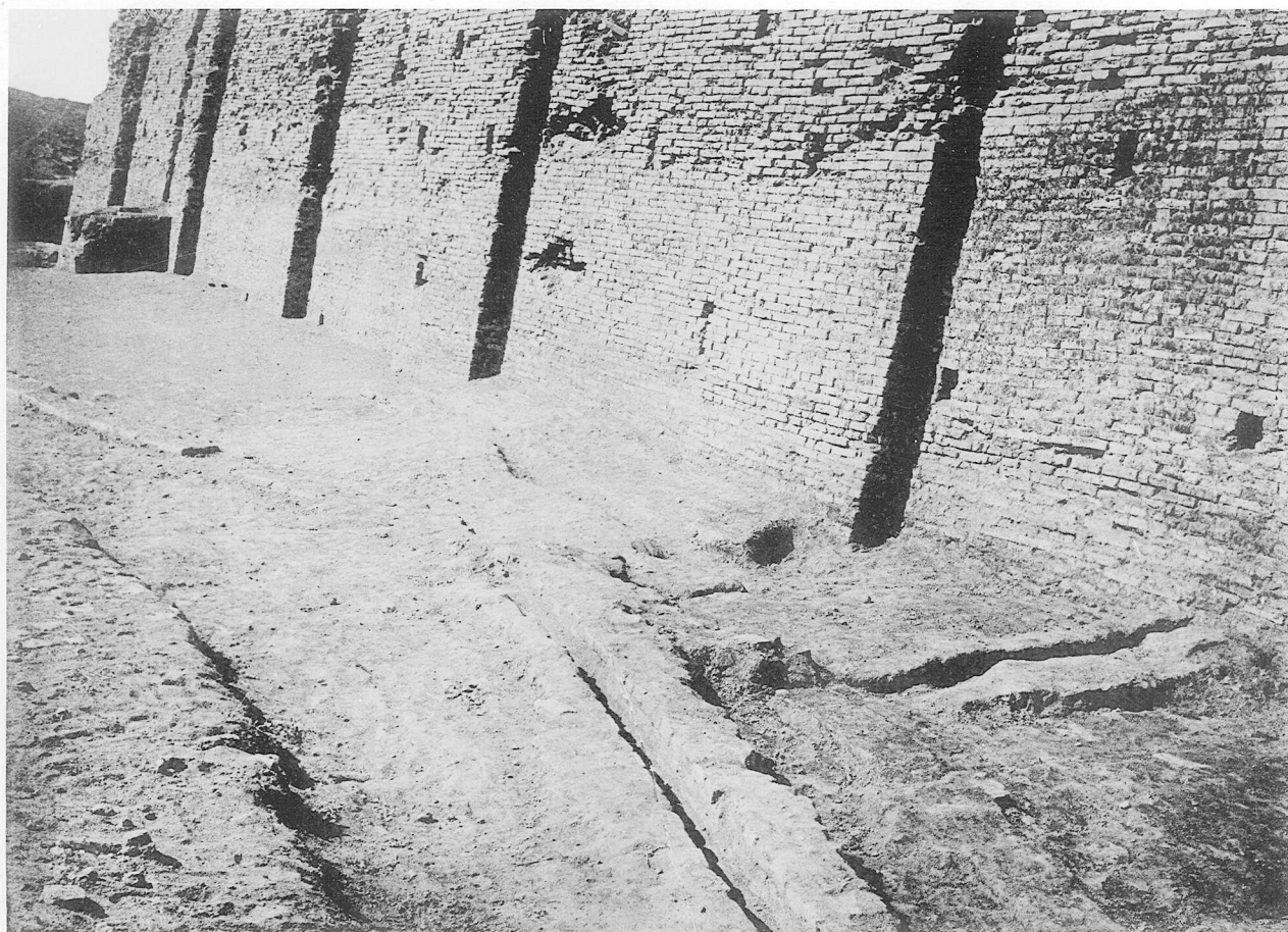
a. The SE. face: E. end, showing late drains. ( See p. 65 )
