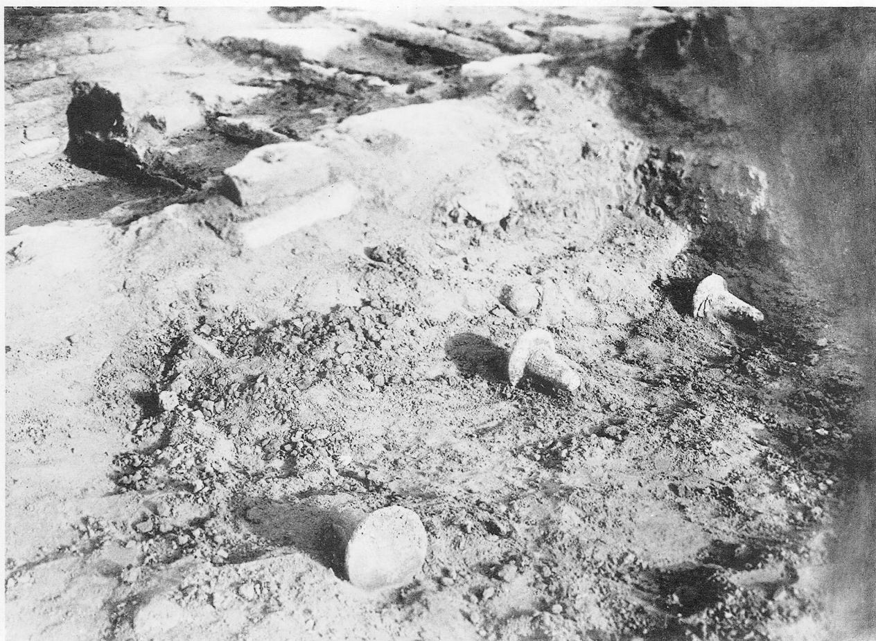
b. The Warad-Sin Bastion: foundation-cones in situ in the core of the wall. (See p. 43)
