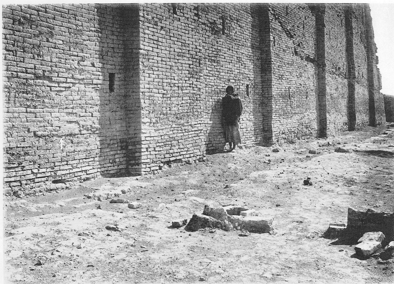
a. The SW. face: the brickwork in the first bay was repaired in Larsa times (stamped brick of Bur-Sin found here). ( See pp. 73, 122 )
