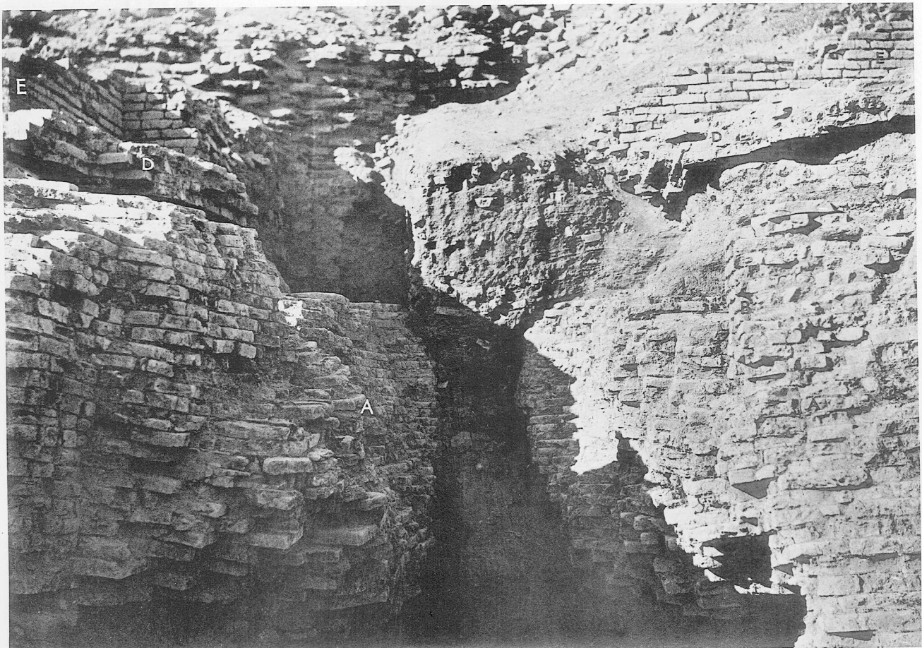
b. Taylor's cut, looking SW., showing: A, A, foundations of Ur-Nammu's upper stairs; B, face of jamb at stair-foot; C, rubbish filling left by Taylor; D, D, Nabonidus' terrace pavement; E, E, Nabonidus' terrace front; F, Nabonidus' mud-brick upper core
