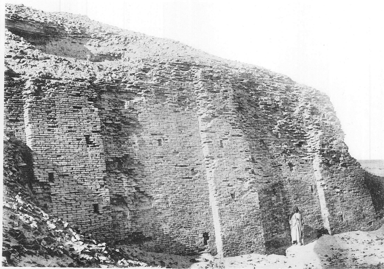
b. The SE. face: the east corner cleared
