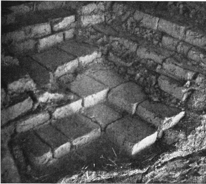
Unburned Bricks of the Tower of Akkerkuf.
