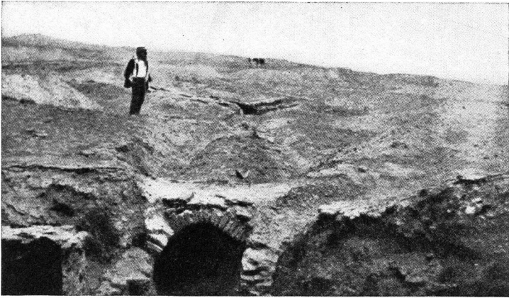
An Arched Sewer of Plano-Convex Bricks.
