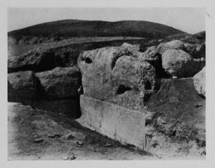
$F_{IG}$ . 29. Ashlar masonry of the south wall of the south-east tower, and the rubble building abutting on it.
