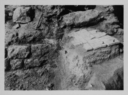
$F_{1G}$ .  $2_3$ . The south-east corner of the Gate-tower. A. Foundations of the flanking tower. B. Stratum of limestone chips made by dressing the stones at the time of building. C. Pavement of mud brick resting on the builders' rubbish. D. Retaining-wall for the talus of the mound.
