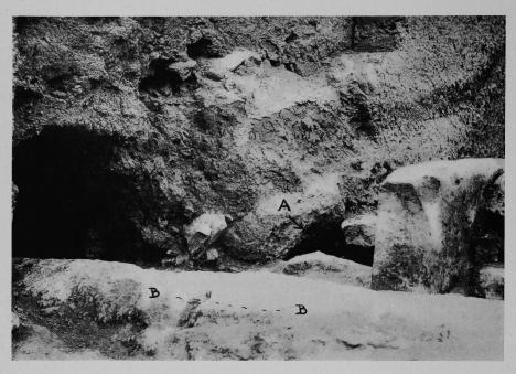
Fig. 16. The blocking-wall in the West Gate. A. The Late Hittite conduit. B. The Roman water-pipe. The wall face was mud-plastered: higher up, the outer skin of bricks has fallen away and actual bricks are exposed.
