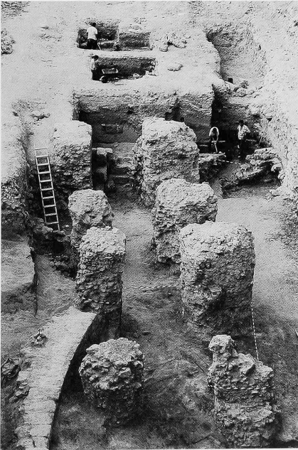
Fig. 4 - College site. Foundation pillars of the school aligned on two parallel lines.
