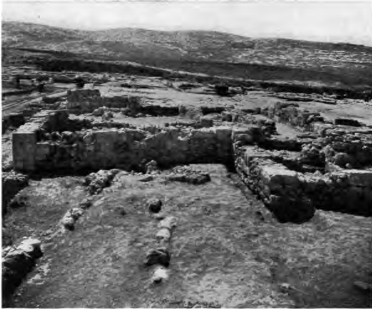
FIG. 23.—The east side of the large house in Stratum IV, from E. (cf. OIC , No. 4, Fig. 43), with the tower on the right. Note the alternation of ashlar with rubble, and of headers with stretchers, in the former.
