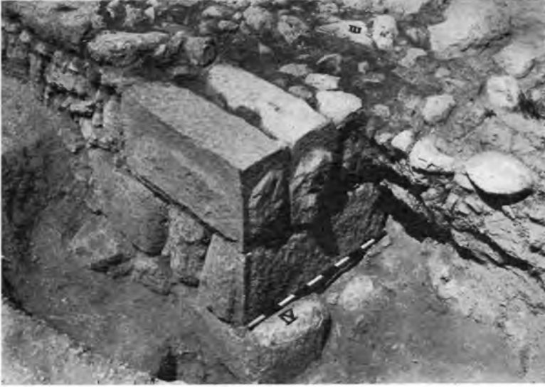
FIG. 31.—The NE. corner of stable No. 403 (cf. Fig. 30). Note the right angle cut in the foundation course, at the near end of the meter stick, to insure the correct positioning of the next stone above.
