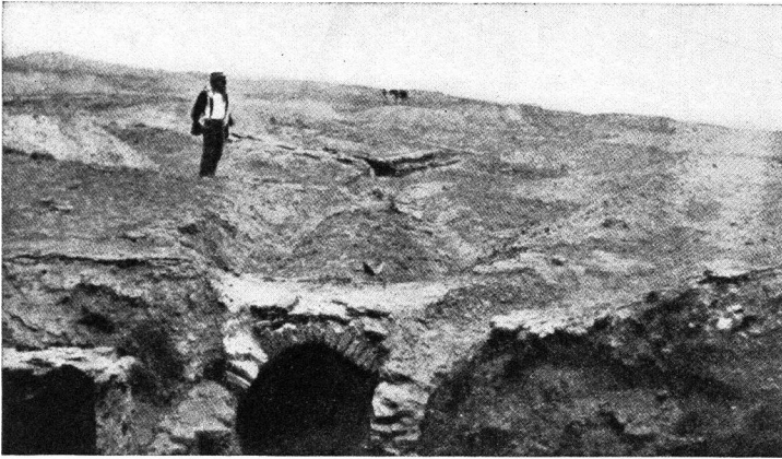
An Arched Sewer of Plano-Convex Bricks.
