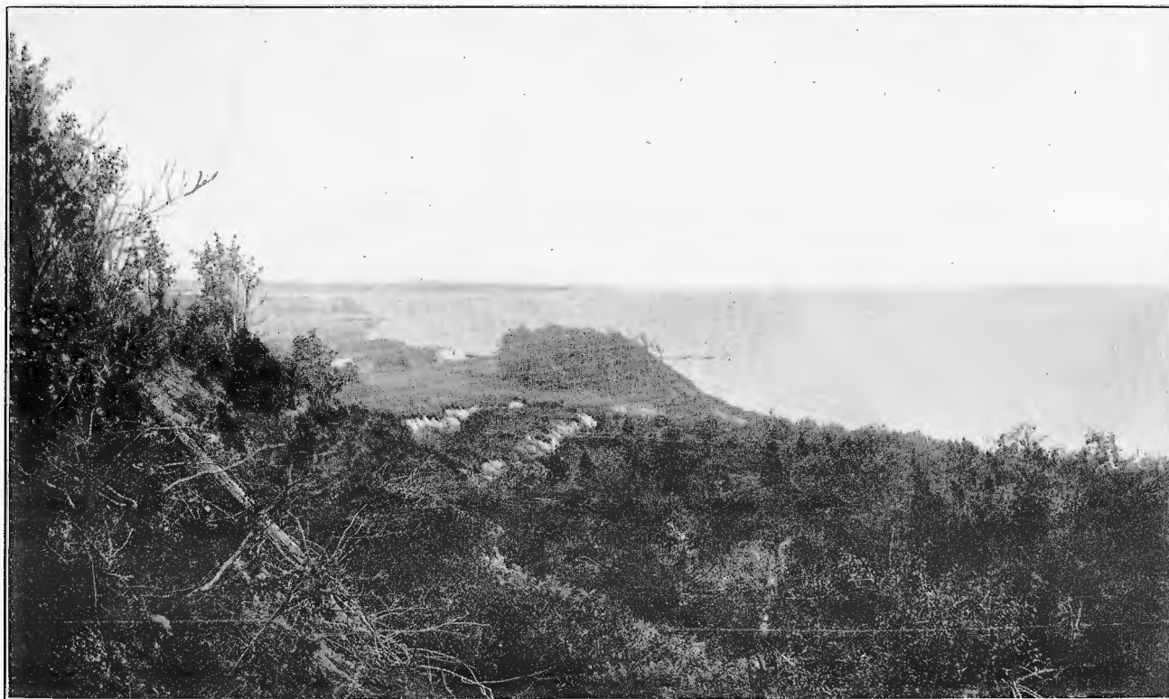
GENERAL VIEW OF GREAT LANDSLIP AREA AT BROKEN GROUND, NORTHEAST OF NORTHPORT.
