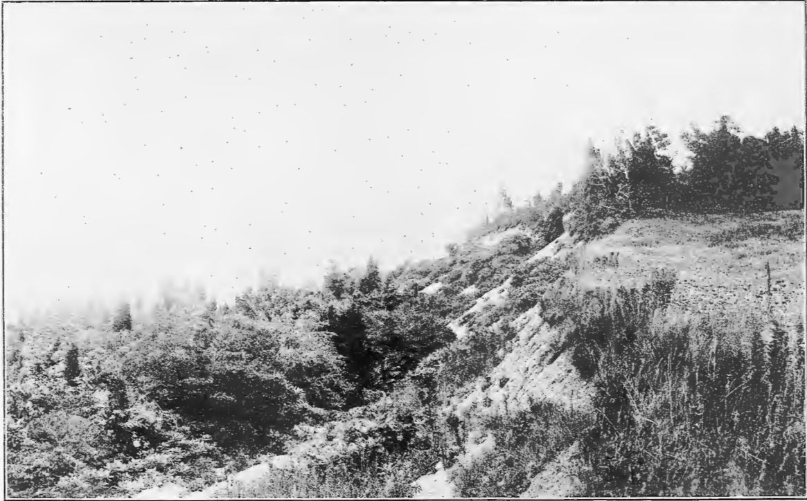
A. MAIN SCARP AT BROKEN GROUND LANDSLIP AREA, NORTHEAST OF NORTHPORT. Photograph by G. N. Knapp.
