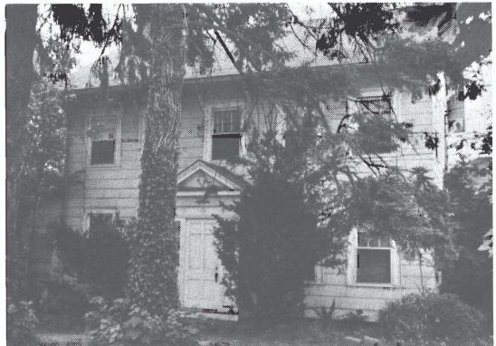
Brush House, Village of the Branch
