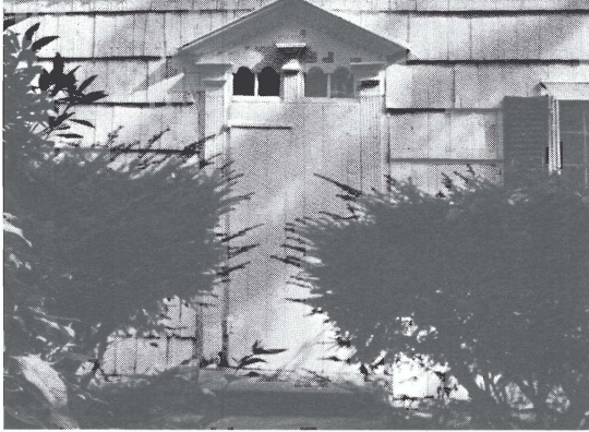
Millard House, Door
