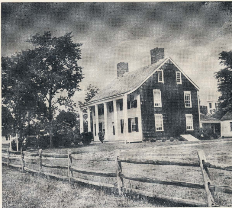
The Webb House at Orient as it is today
