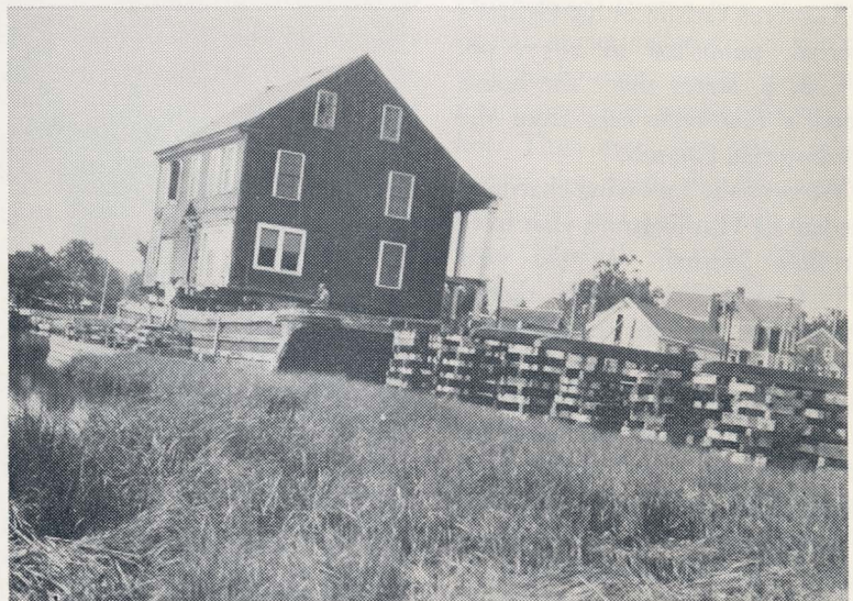
Getting the house on a barge was a complicated process. Note the elaborate cribbing for raising the house to the deck.
