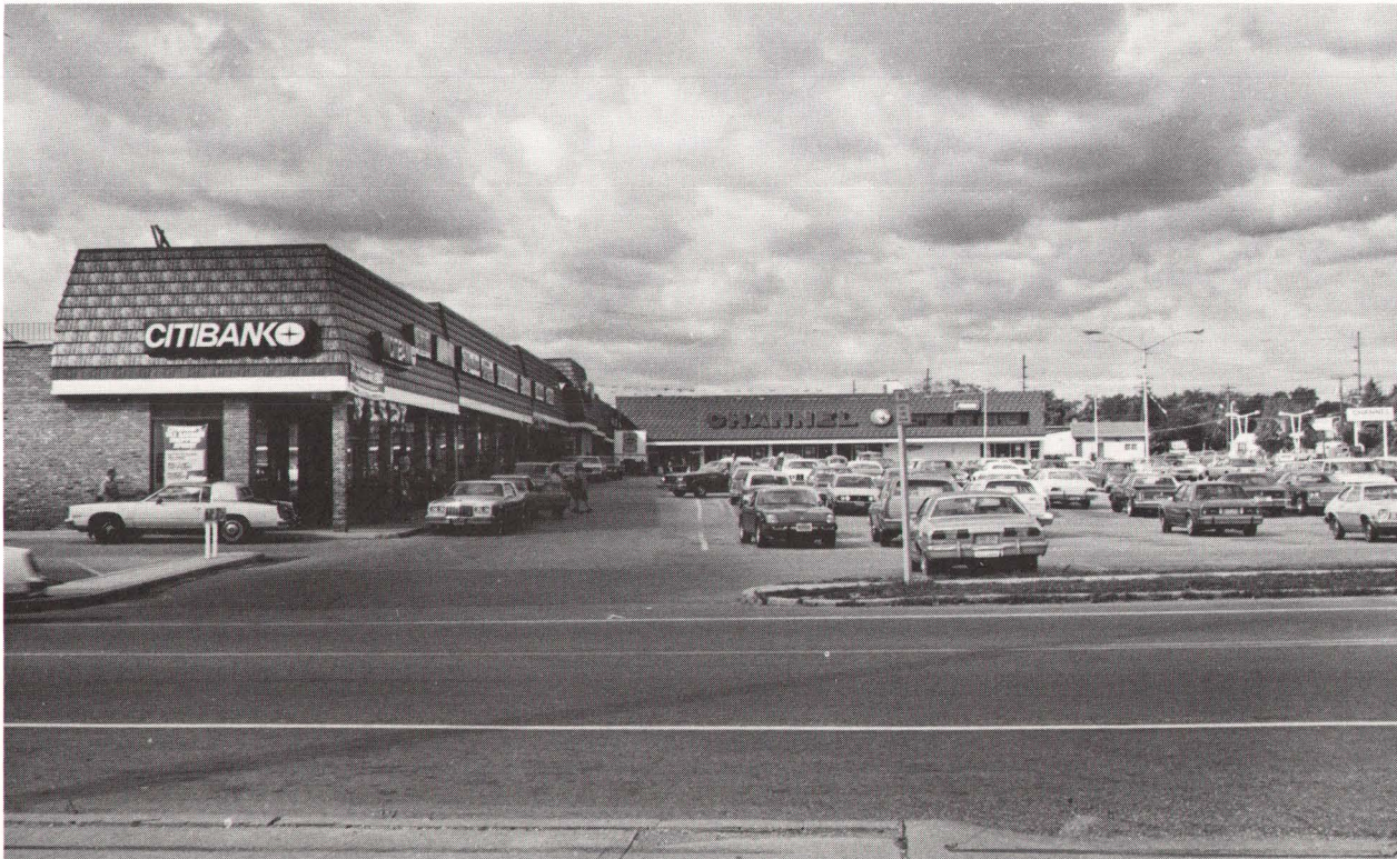
2. North Massapequa Typical neighborhood shopping center.
