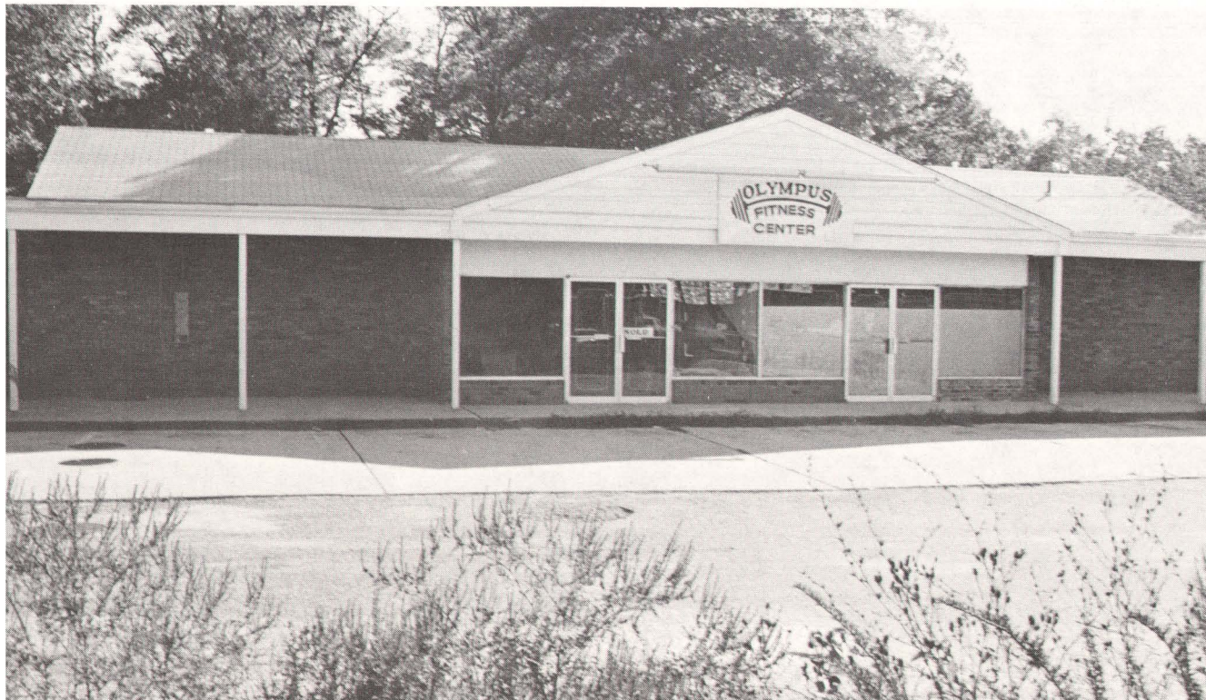
26. East Northport Convenience store converted to a health facility.
